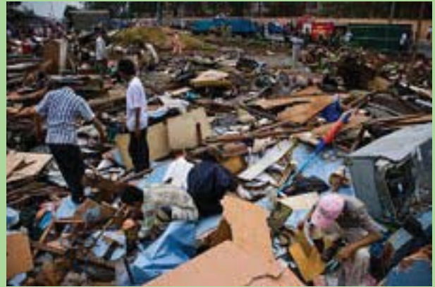
People search through the rubble of their homes after the Dey Krahorm settlement was demolished by police and private 'breakers'.
